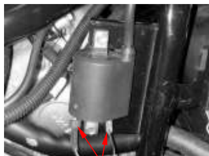
First circuit coil resistance measurement
